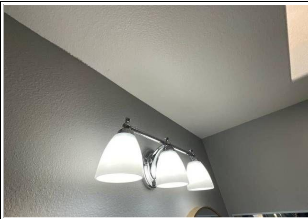
BATHROOM 3 TRACK LIGHTING
