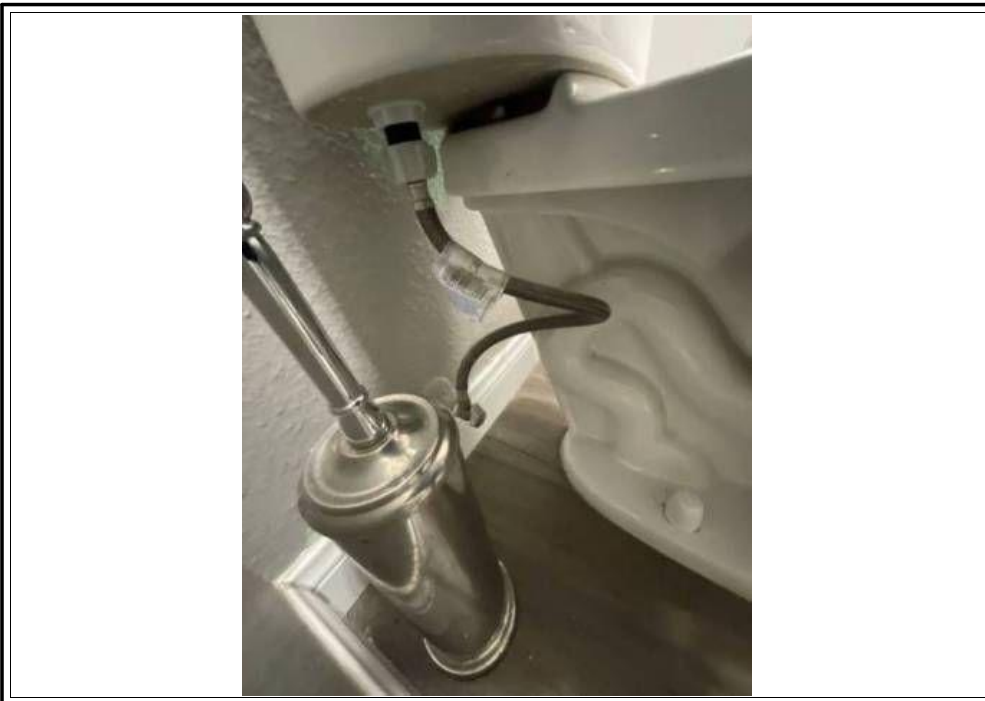
BATHROOM 1 NEW PLUMBING LINES
